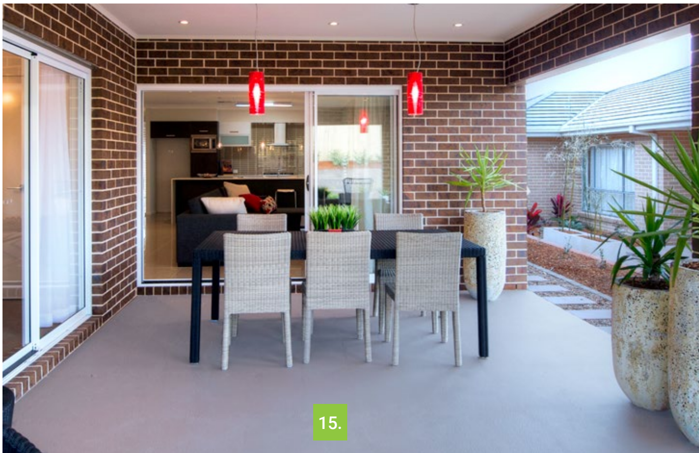
15. SCREED CONCRETE FLOOR TO ALFRESCO Screed concrete finish to alfresco floor.
